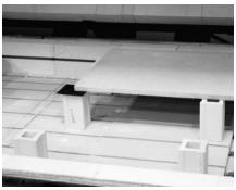
Figure 5: stainless steel shim inserted to raise a low corner.
