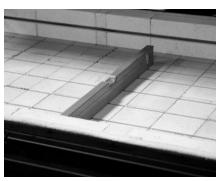
Figure 2: Checking the kiln floor with a level.
