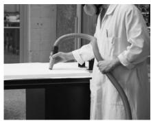
*Figure 10: vacuuming dust from the shelf after sanding.*
